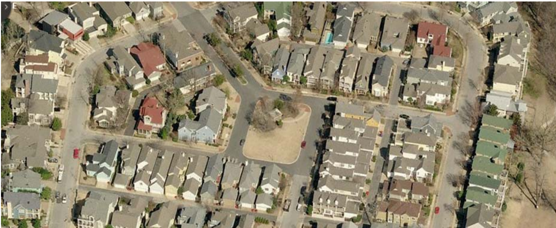
This aerial view of Harbor Town in Memphis, Tennessee illustrates pedestrian oriented development: 1) designated civic space, 2) access by alley, 3) buildings brought up close to street, and 4) higher density
